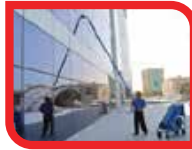
Glass cleaning Exterior & Interior
