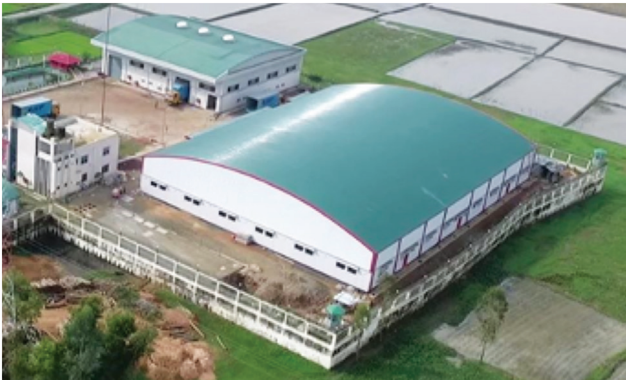
Aerial view of warehouse
